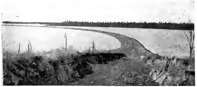
Dyke which diverts Falcon River.
